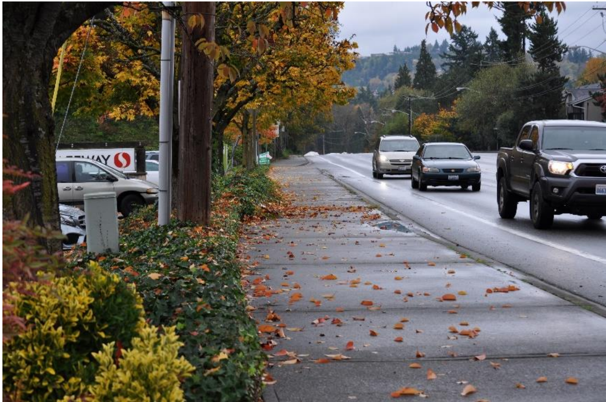
Exhibit 15. Sidewalks on Coal Creek
